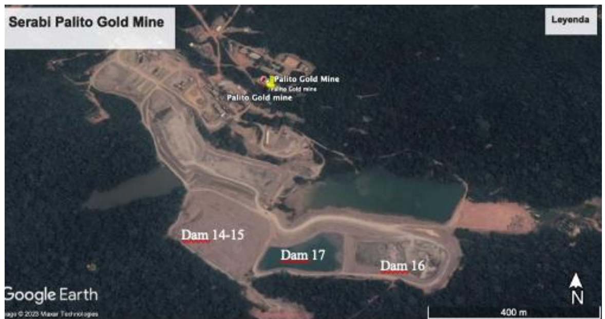
Figure 18-5: General View of Tailings Dam Area
