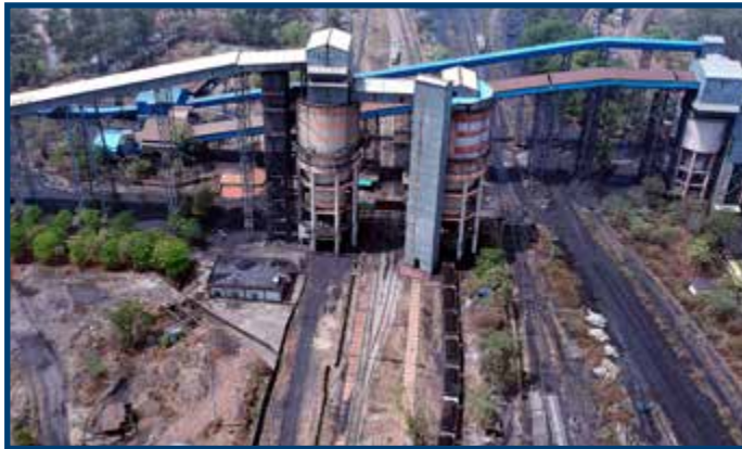
Rapid Loading System-SILO at Gevra Area
