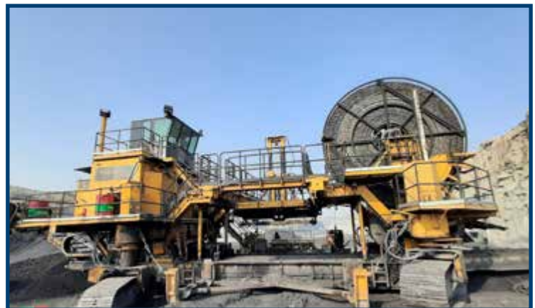
Highwall Operation at Sharda Mine, Sohagpur Area
