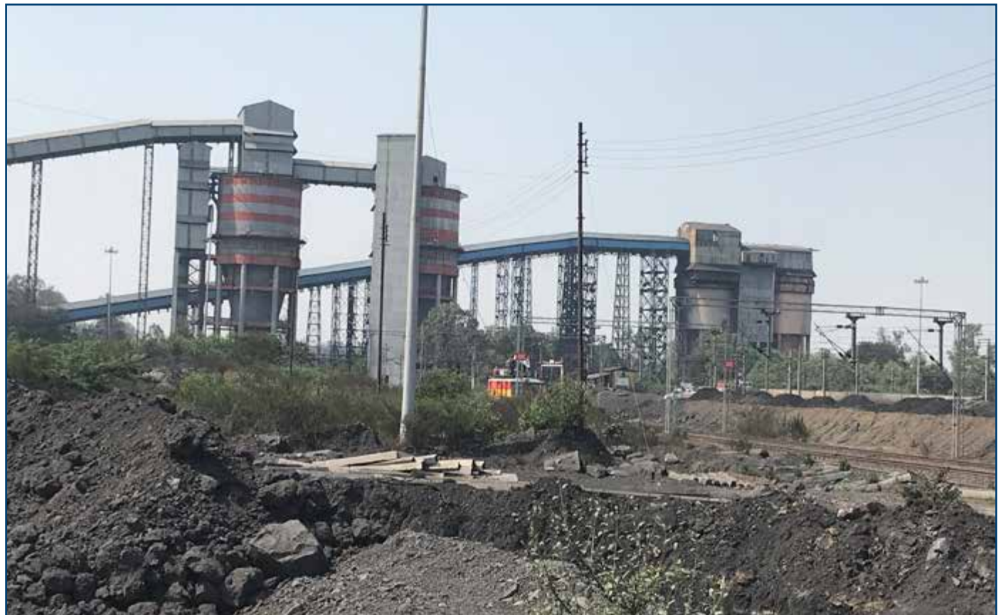
Rapid Loading System (SILO) at Gevra Area (Old & New)
