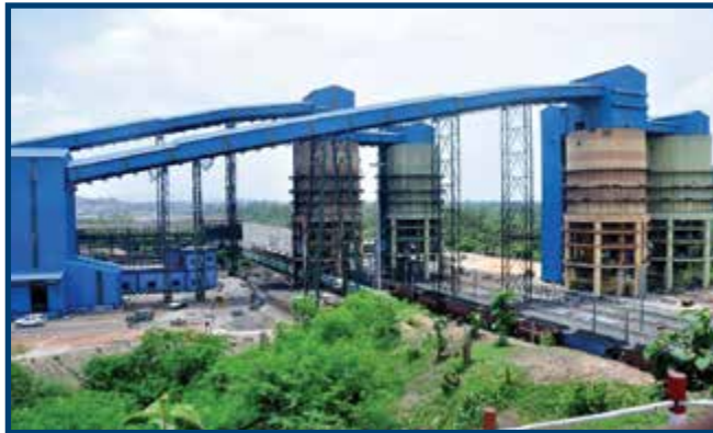
Wagon loading through SILO at CHP, Kusmunda OC
