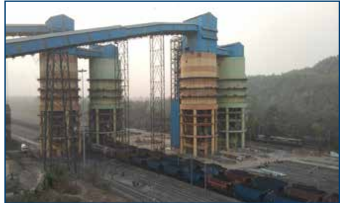
New 04 Nos. of SILO at Kusunda Area based on Pre-Weigh System
