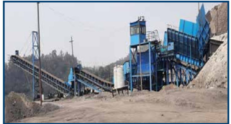
1000 THP Semi Mobile Crusher at Gevra OC
