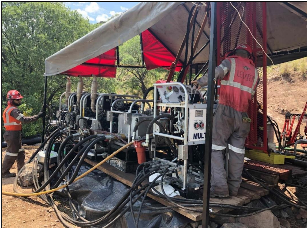
Figure 10-1: Man-Portable Drilling Rig at Site of SJ21-01
