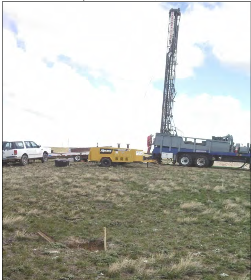
Figure 13. Photo of URE Confirmation Drilling
