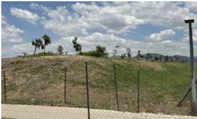
Trees were recently relocated and planted along PCD to construct a mitigation measure berm
