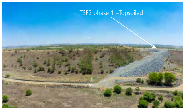
TSF 2 phase 1 – Topsoil and revegetation in progress
