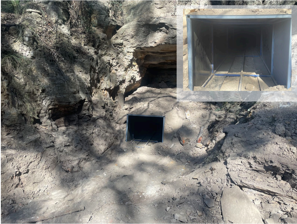
Photo 2 Upgrades to the Bat Adit Culvert in 2023
