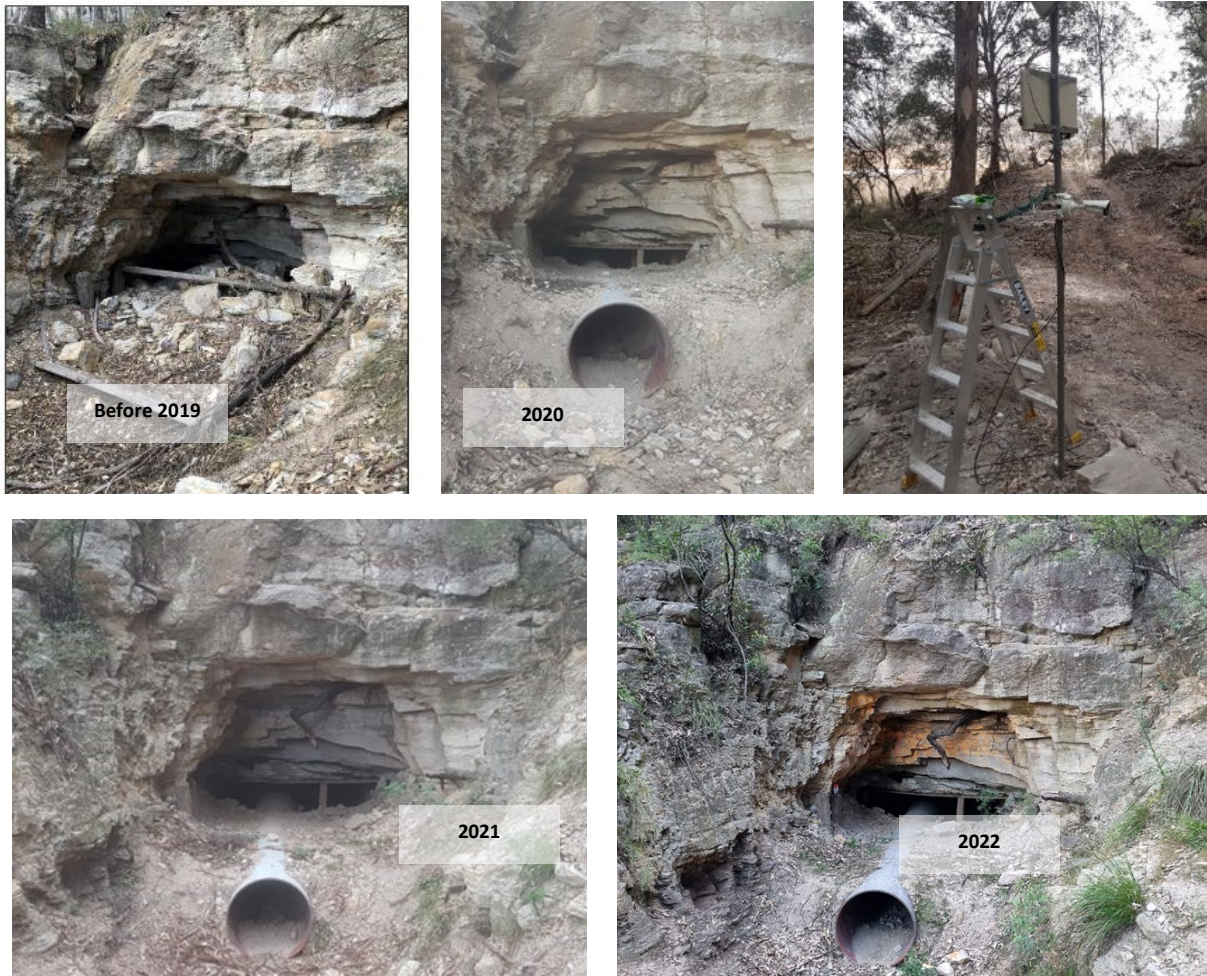
Photo 1 Culvert Support & Bat Detector with Solar Panel setup 20m in front of Adit
