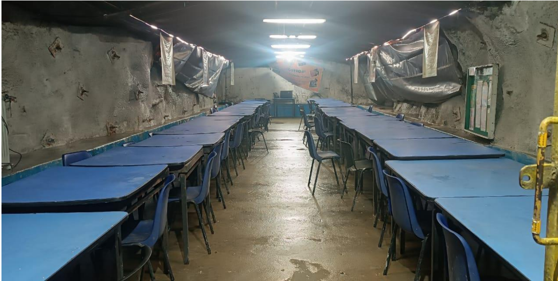
Figure 18-7: Yauricocha NV 1070 Crib Room
