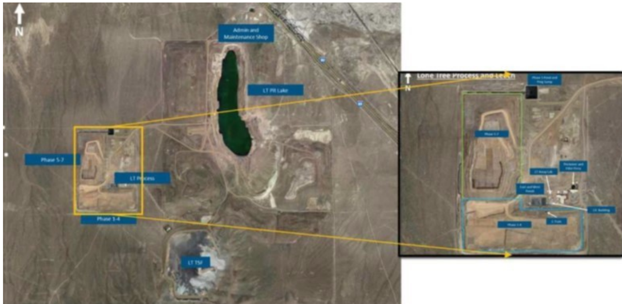
Figure 1-2: The Location of the Lone Tree Deposit and Infrastructure
