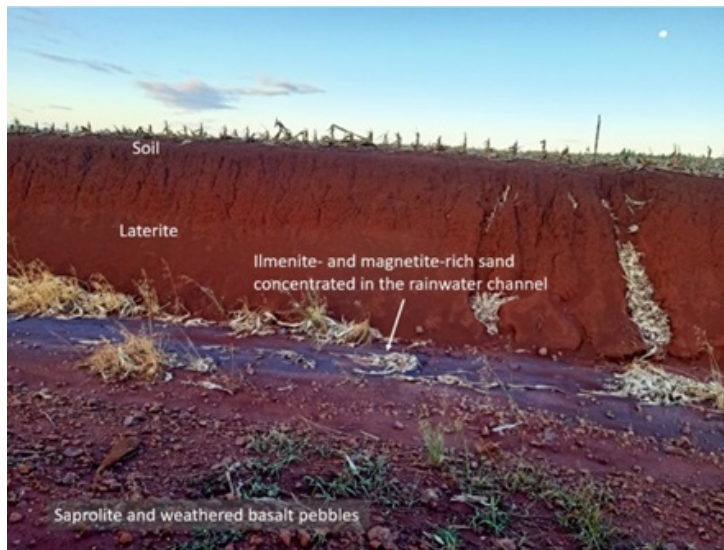
Figure 6-10: Road cutting at Block A showing the laterite profile
