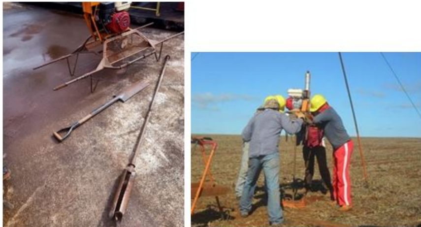
Figure 7-3: Mechanized auger for drilling deeper auger samples
