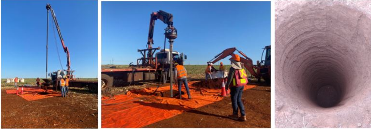
Figure 11-4: Large diameter auger drilling bulk density test
