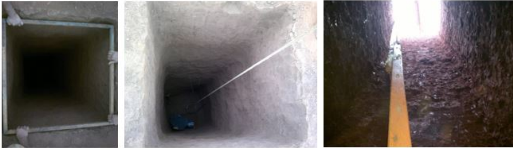
Figure 11-3: Bulk density determination by pit excavation (2011)
