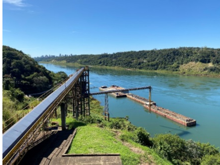
Figure 15-4: Barge loading port on the Paraná River
