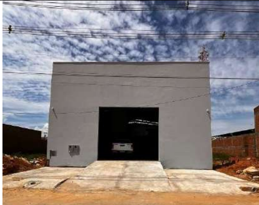
Core Shed House 3 of the Lithium Ionic in Araçuaí-MG-Brazil – external view
