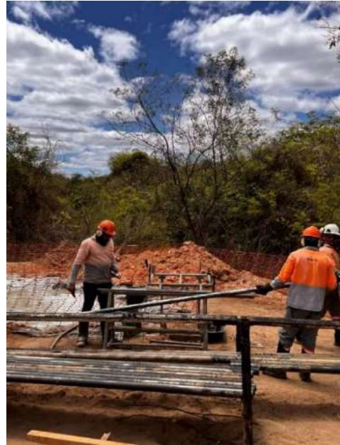
Drill Rig on site of the Bandeira, drilling in 13/09/2023 – DDH ITDD-23-192 - Technicians recovering the cores and using the REFLEX ACT III for core orientation
