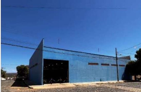
Core Shed House 2 of the Lithium Ionic in Araçuaí-MG-Brazil – external view
