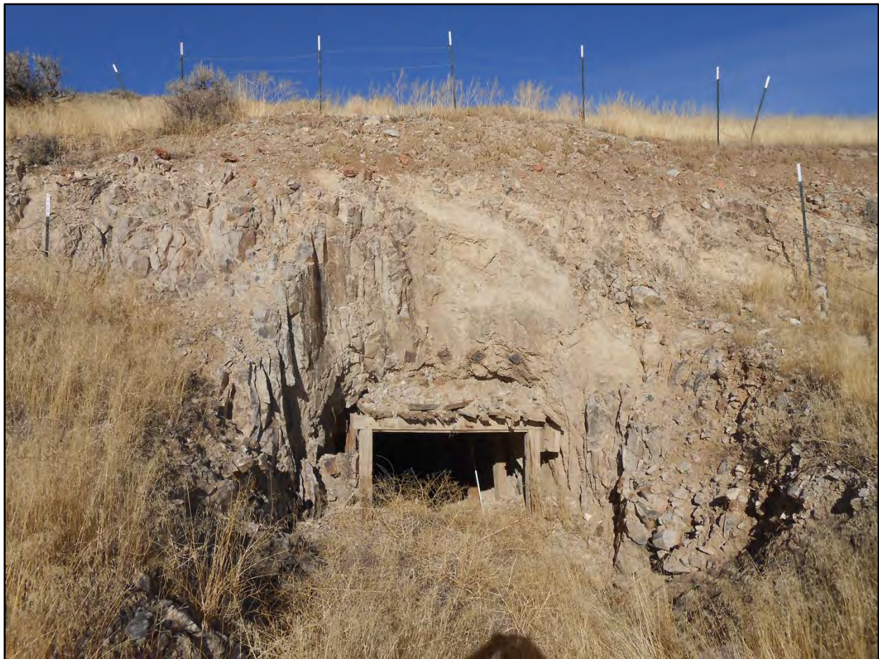
Figure 7.12: Sphinx Decline Adit
