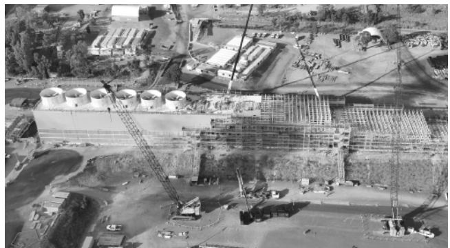
New C4 cooling tower construction as of end of June 2024.
