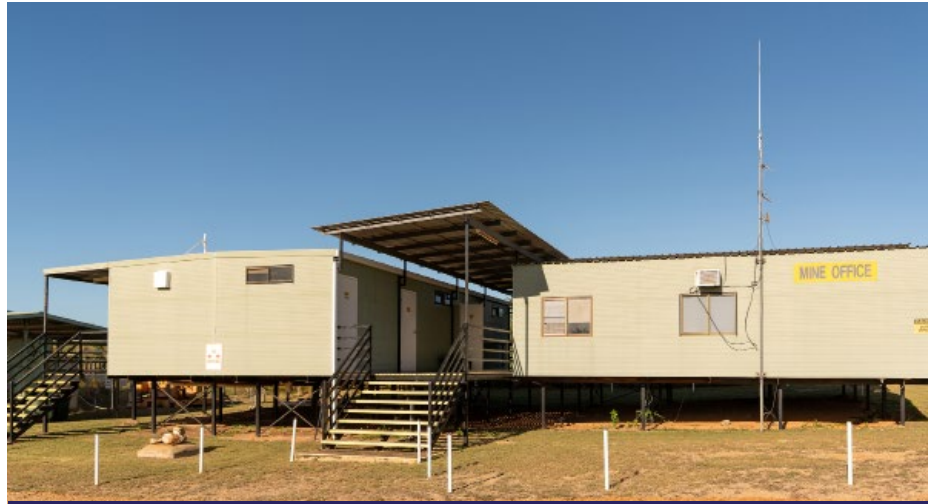
2 Mine Site Office
