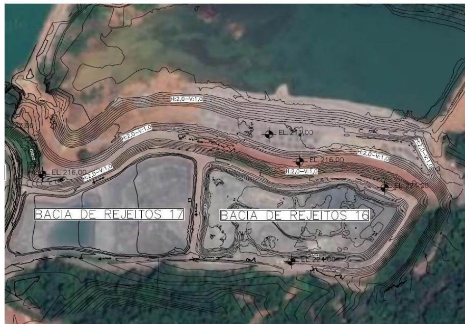
Figure 18-2: Active Tailings Dams 16-17
