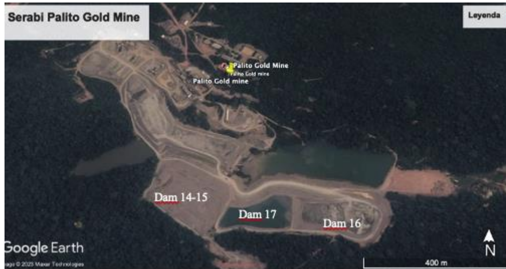
Figure 18-3: General View of Palito Tailings Dam Area
