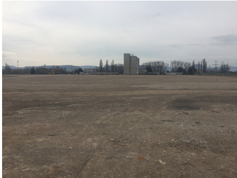
Figure 1: EPR1 site in March 2024 after demolition, clearance and ground rehabilitation. The administration building on the west of the site has been retained and is suitable for use as construction offices.
