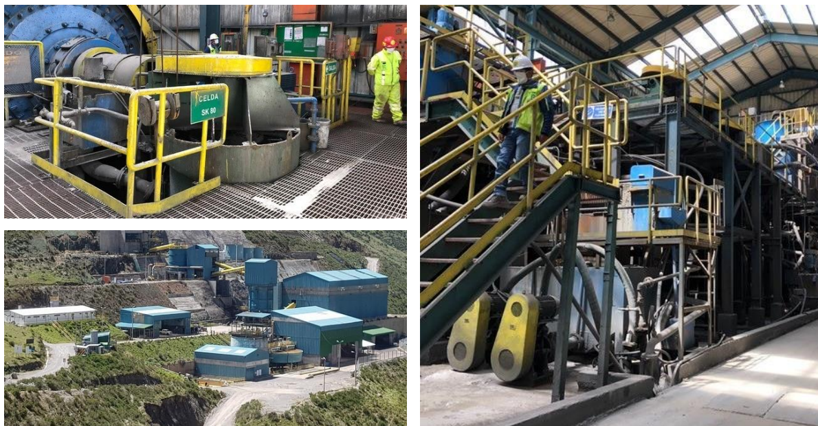
Figure 1: Mally Mine Processing Facilities and Surface Infrastructure
