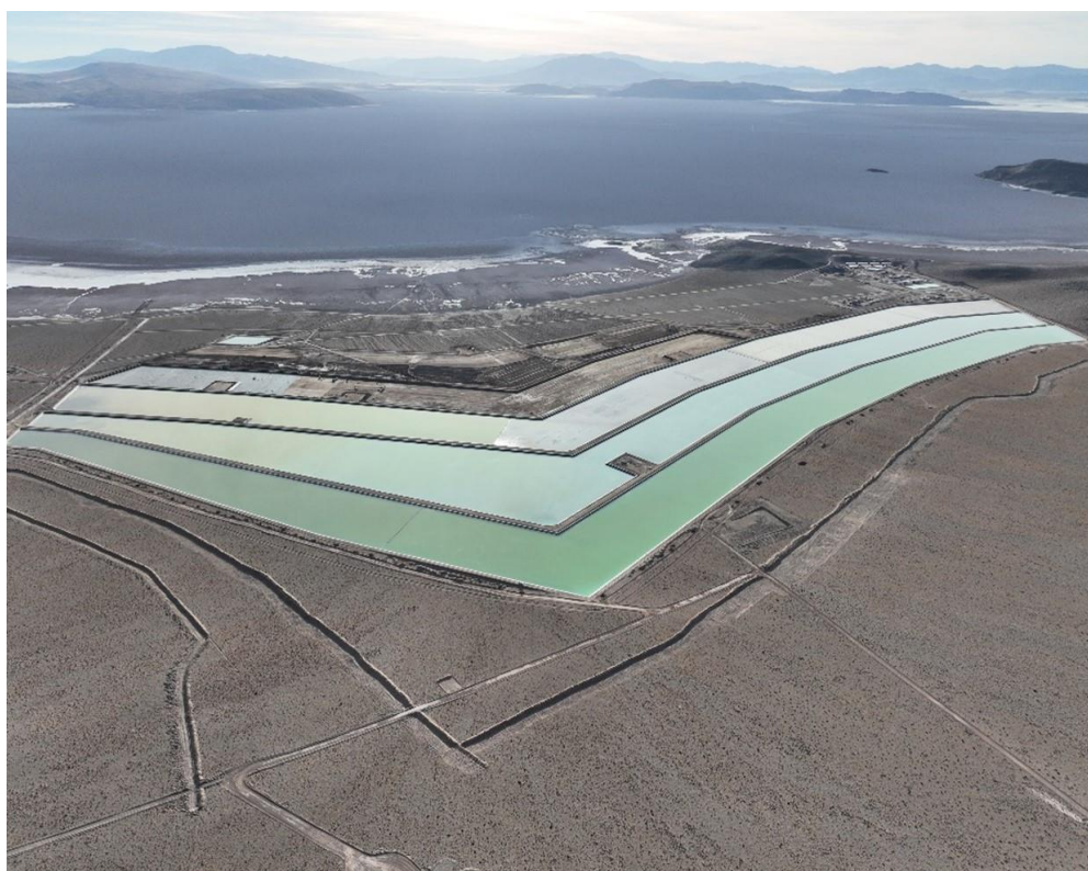
Figure 2. First 3 ponds completed, filled and evaporating
