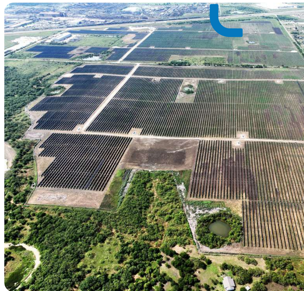
Midlothian solar farm, USA
