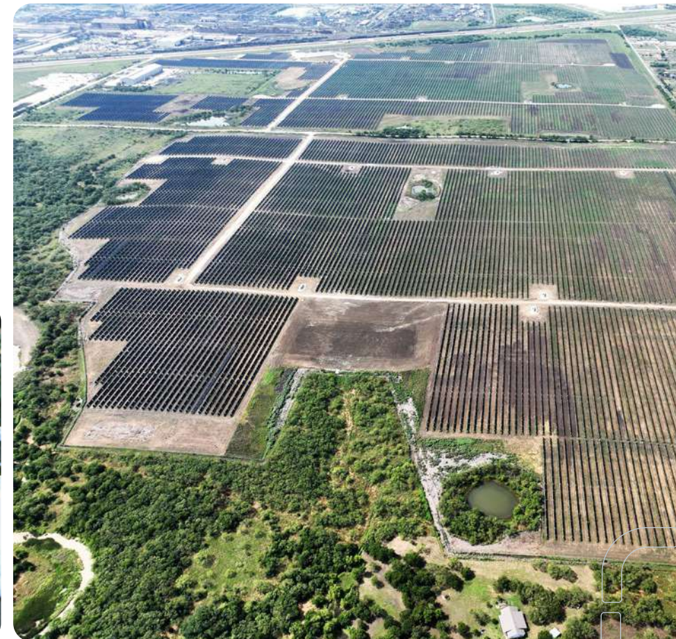
Midlothian solar farm, USA
