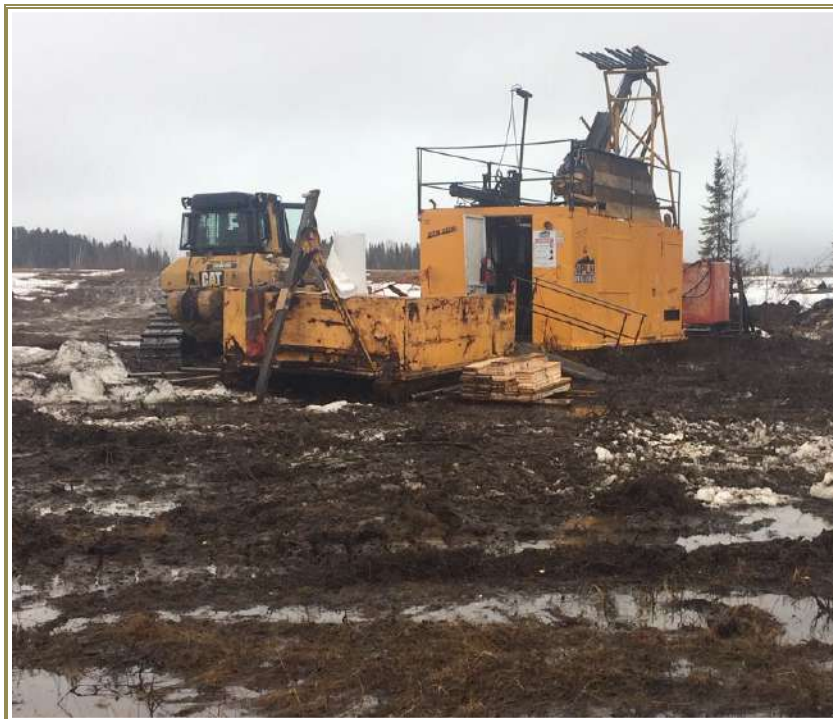
Figure 10-6: Diamond Drill Rig
