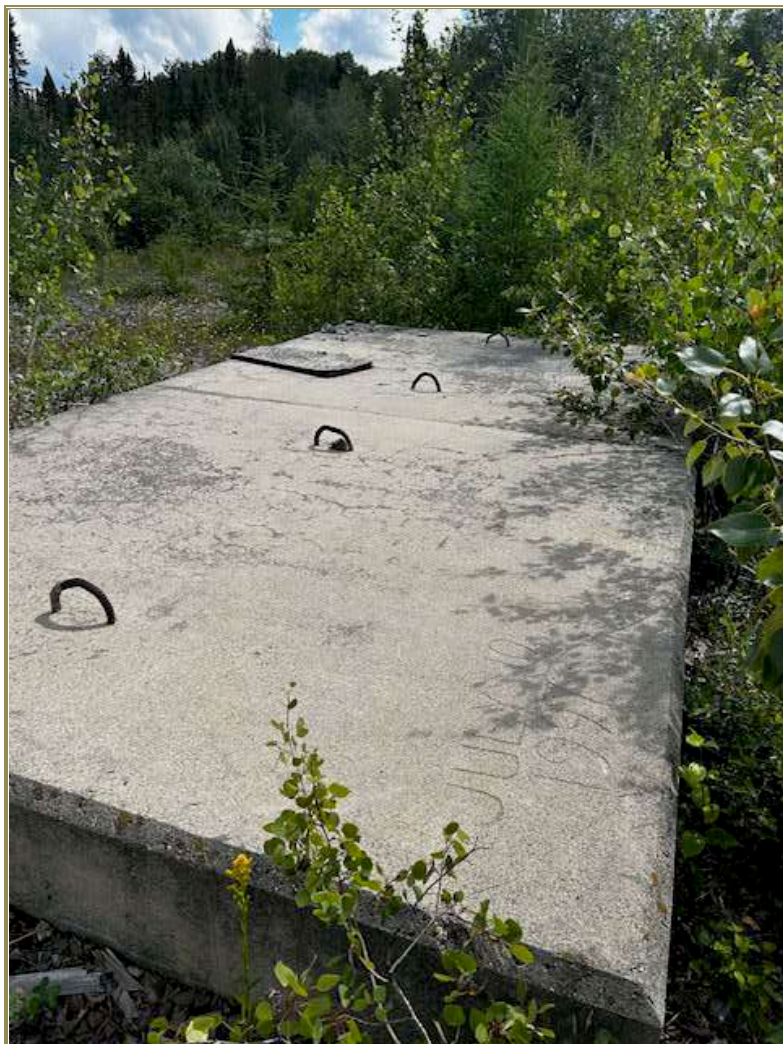
Figure 12-14: Mine Workings—Capped Jellicoe Shaft, Key Lake Property
