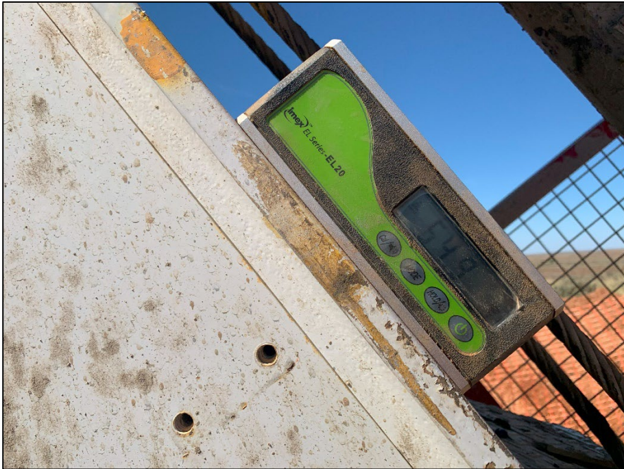
Figure 4: Imex EL20 inclinometer use to determine mast dip angle.
