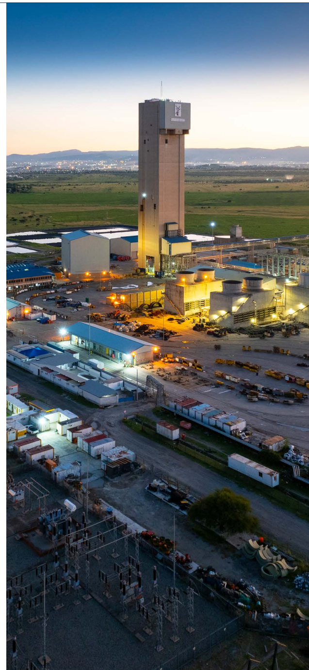
16 Shaft operation at Impala Rustenburg
