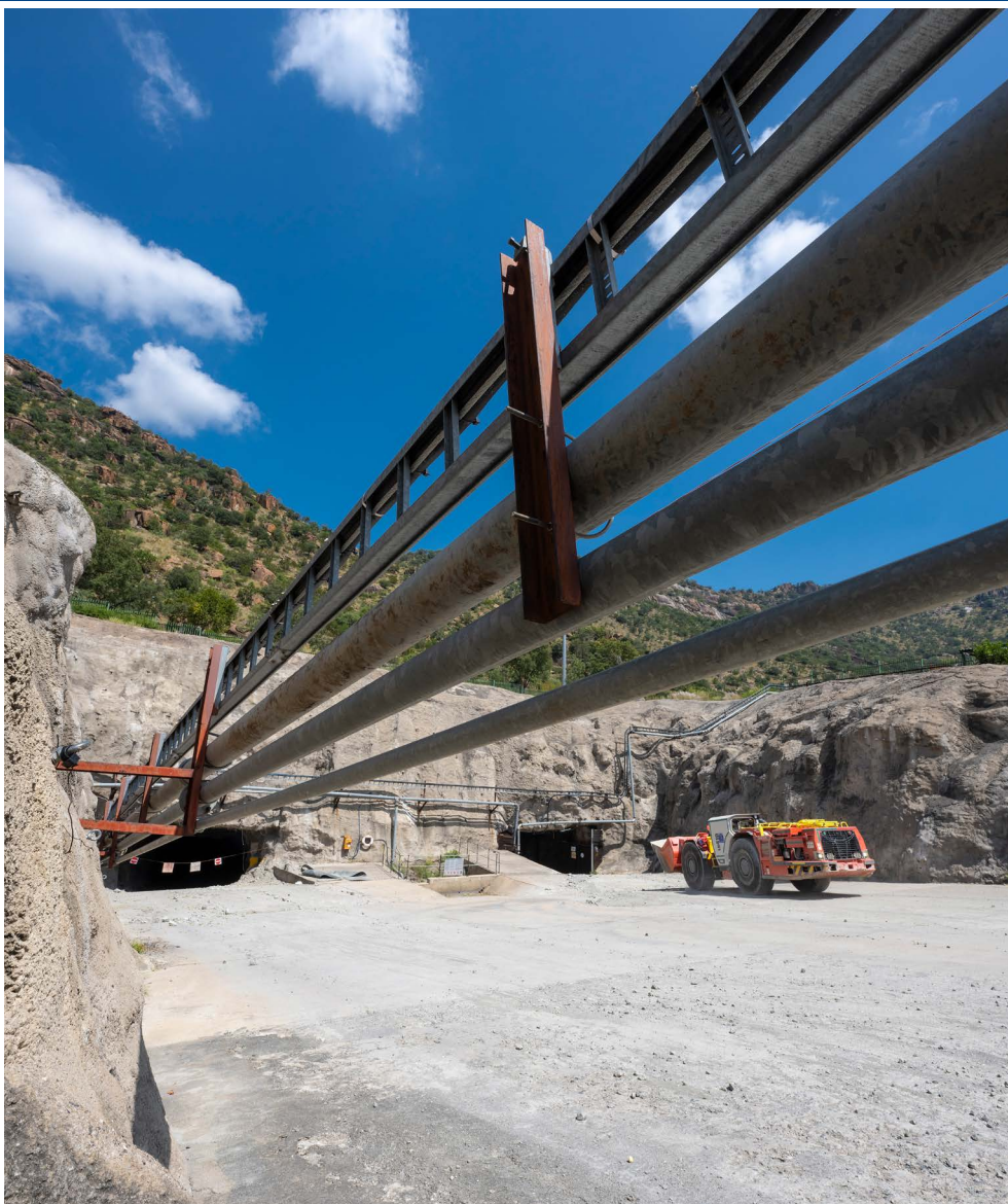
The portal to the decline of the Merensky Shaft at Two Rivers
