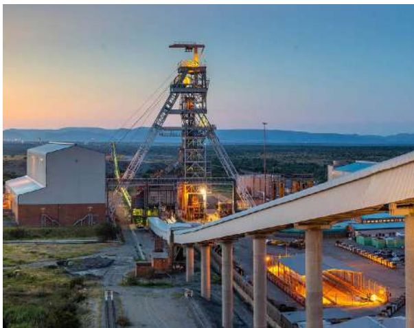
14 Shaft, Impala Rustenburg
