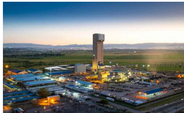
16 Shaft operation at Impala Rustenburg
