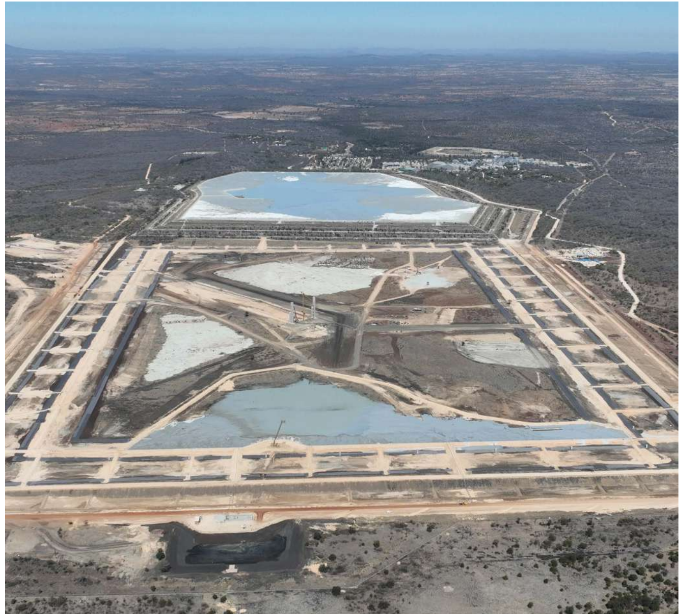
TSF4 at the Mimosa operation
