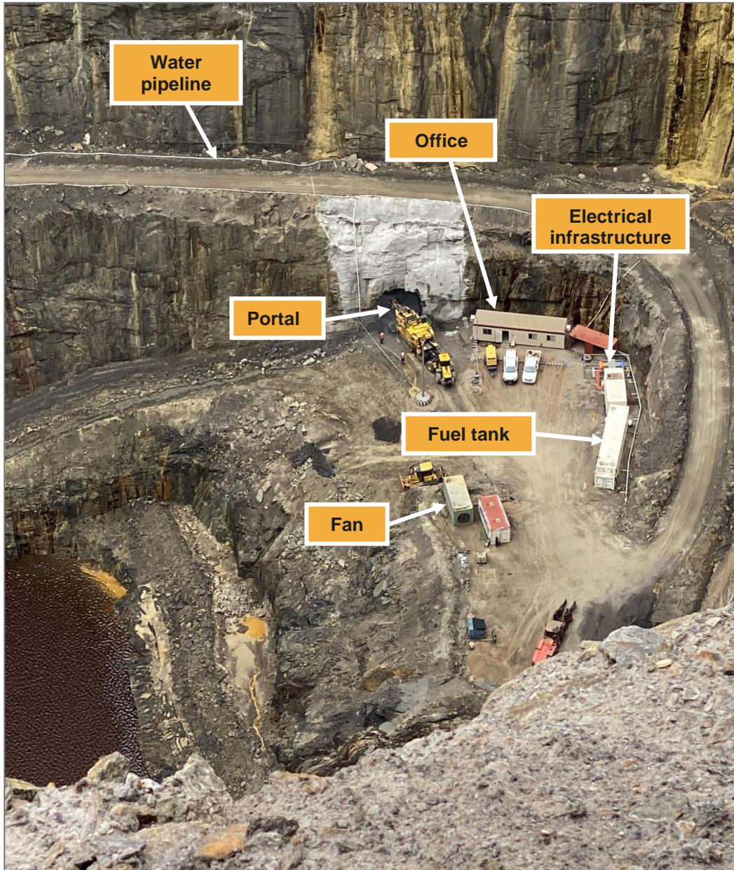
Figure 52: Infrastructure located at the underground portal
