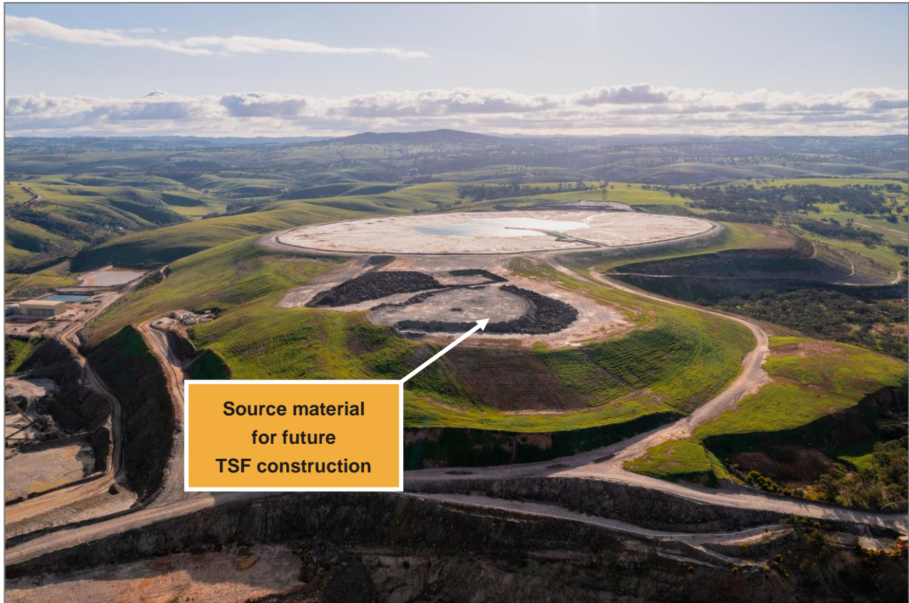
Figure 48: Integrated waste landform showing rehabilitated areas and open areas containing waste rock for future TSF construction
