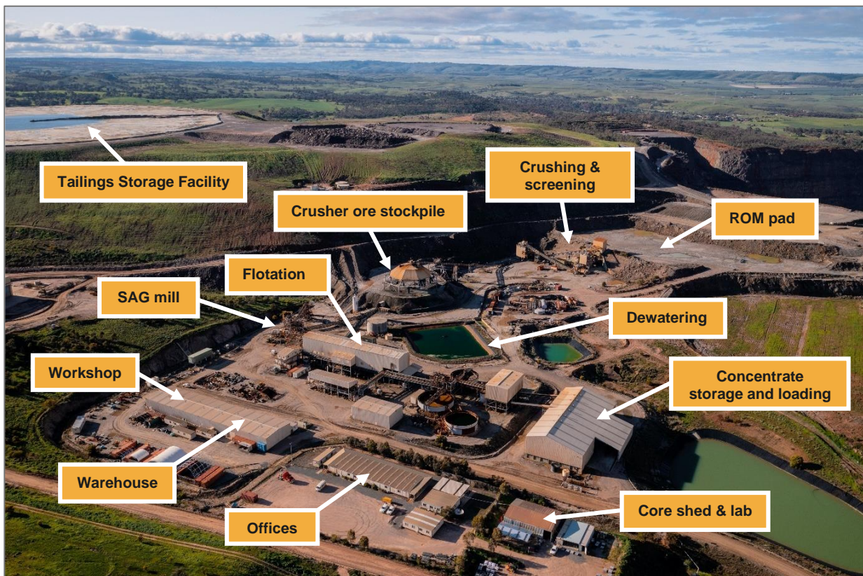
Figure 40: Kanmantoo Copper Mine processing plant and workshops
