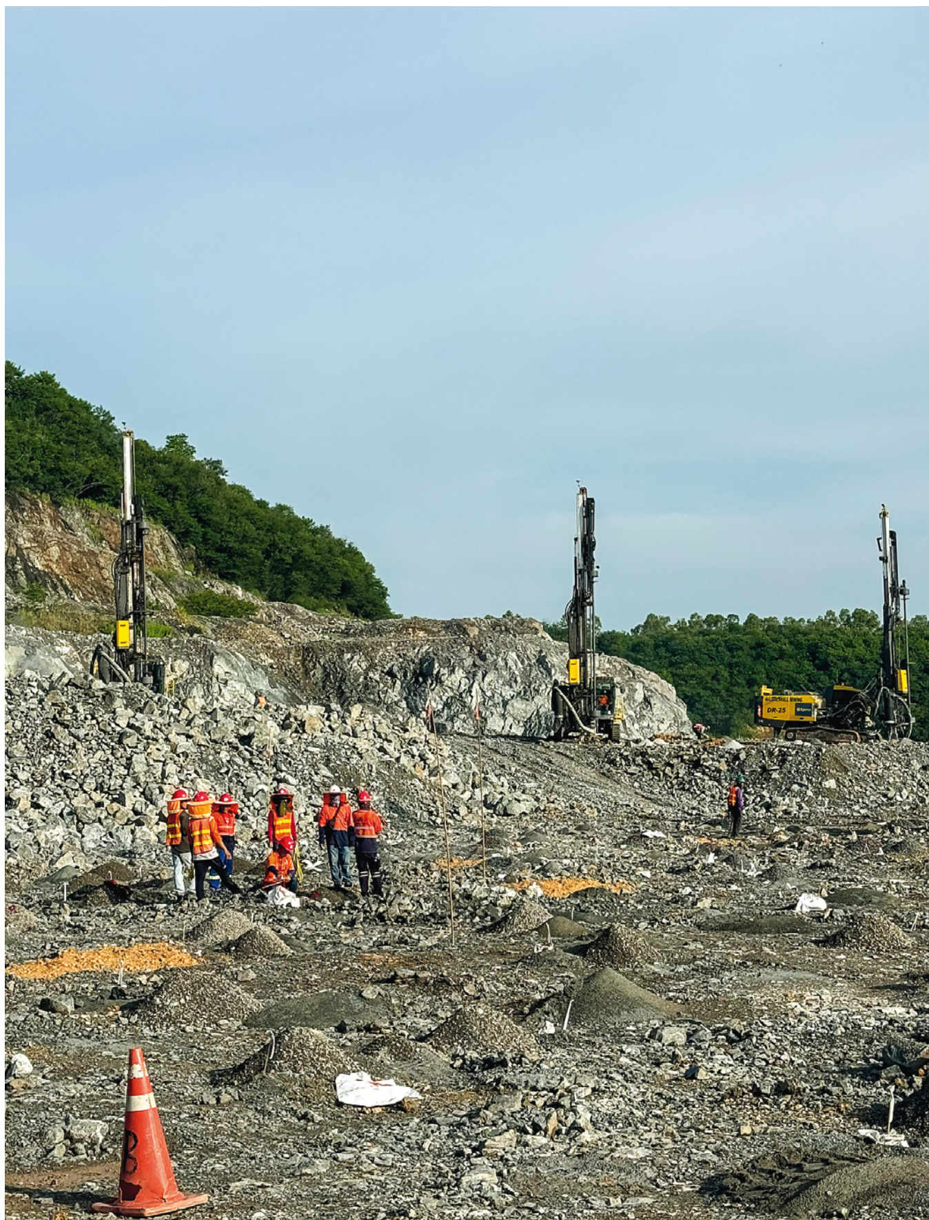
Drill and Blast – A Pit
