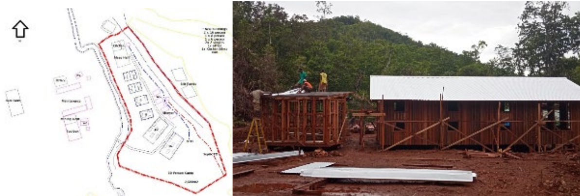
Figure 34 Initial 50 Person Camp Facility
