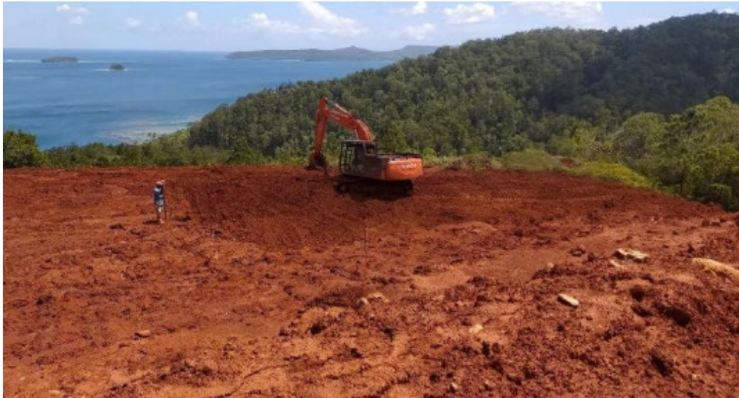
Figure 38 Pit Clearing and Access
