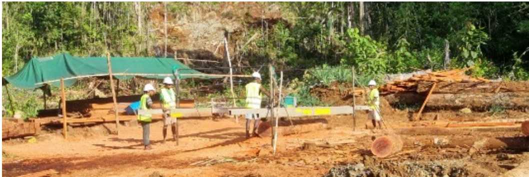
Figure 39 Local Timber Milling On Site
