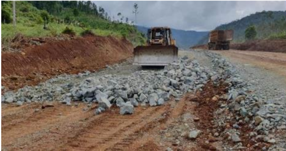
Figure 37. Example – Ni Ore Access & Haul Road Development
