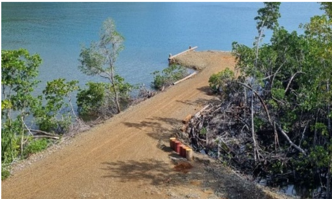
Figure 40 Equipment Landing Wharf
