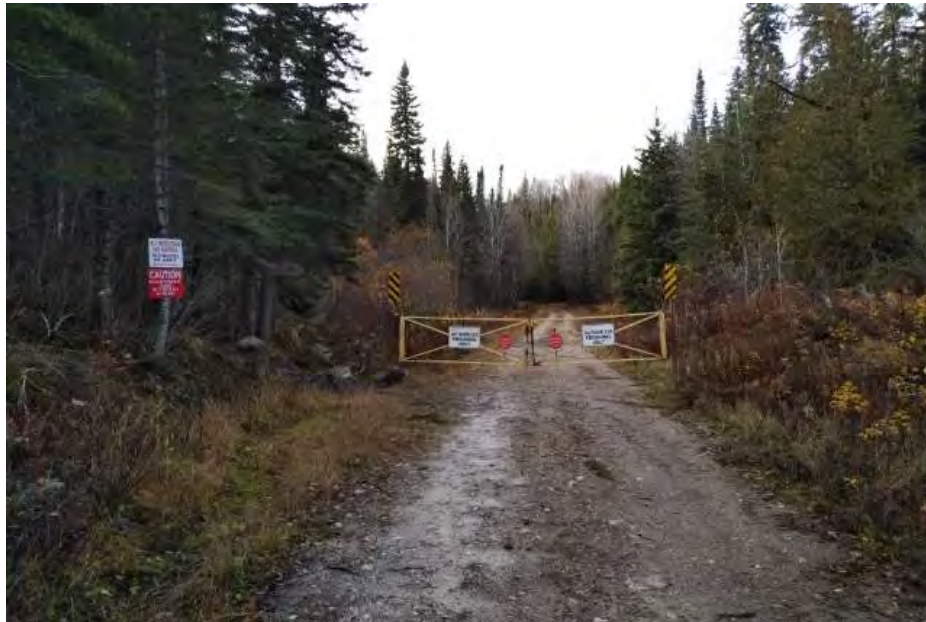
Figure 5.1 : Access Road Photograph
