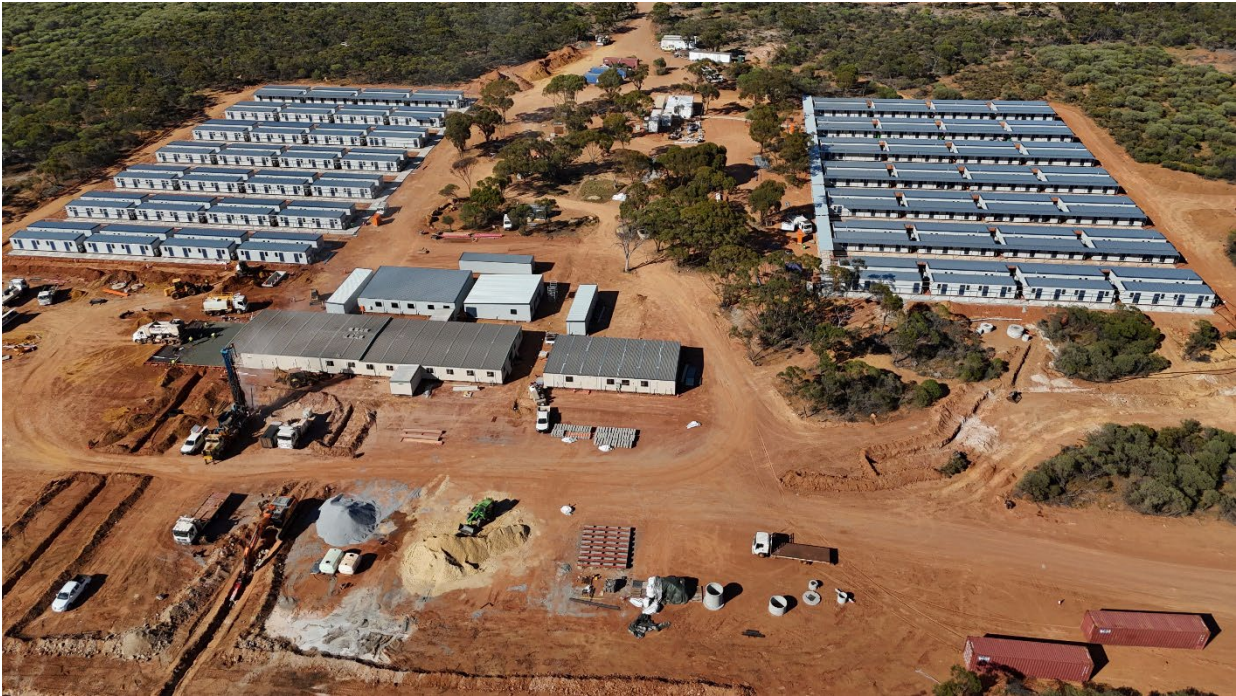
MGGP accommodation build nearing completion.
