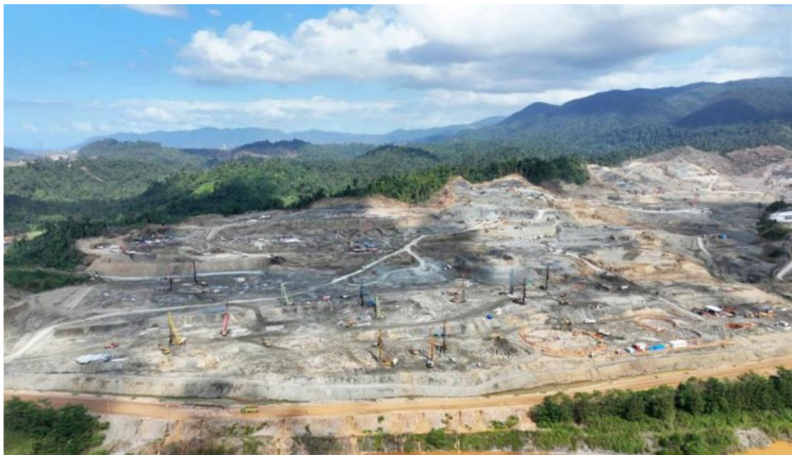
ENC Project under construction
