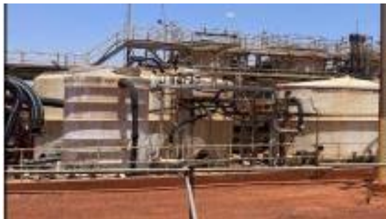
Figure 4 – Solvent Extraction Plant
