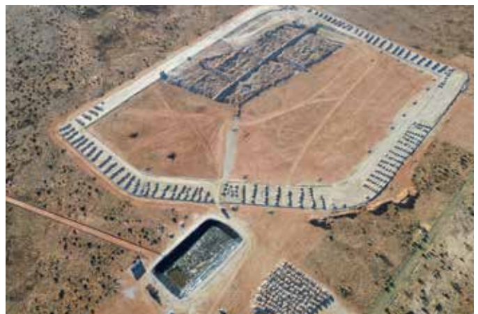
Figure 2: Construction of 13ha Water Storage Dam on 65ha TSF footprint.
