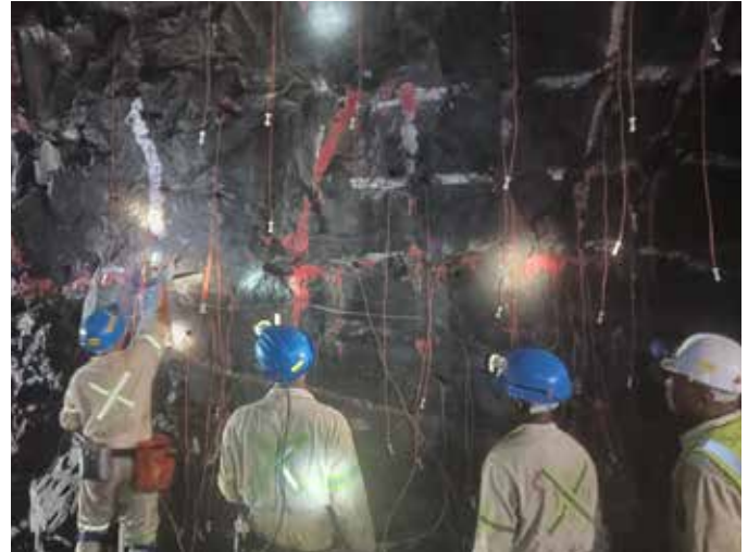
Photo 6: +105 Level face charging.
