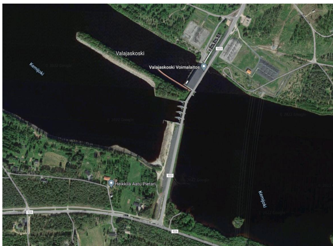
Figure 18-4: Valajaskoski hydroelectric power station
