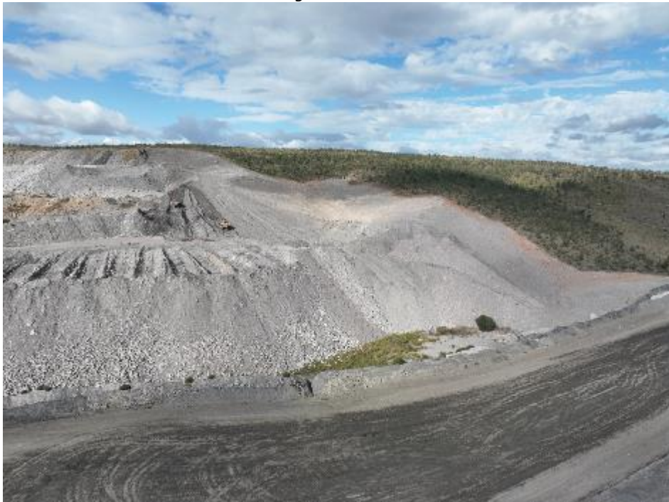
Photo 2 – Rehabilitation Progress 2023. 7 South Rehabilitation Area
