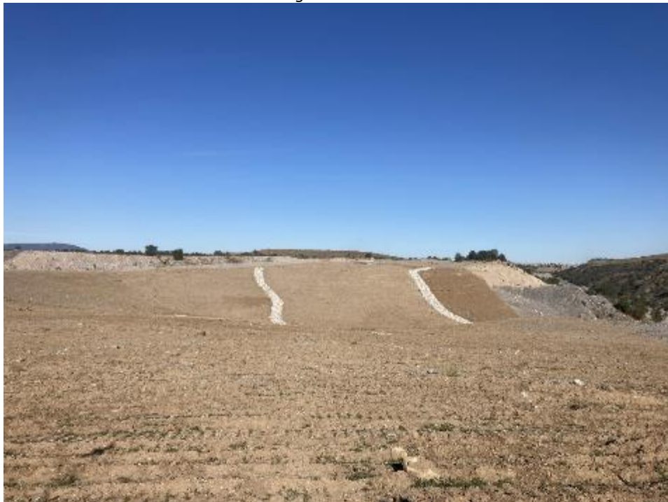
Photo 4 – Rehabilitation Progress 2023. 9 South Rehabilitation Area
