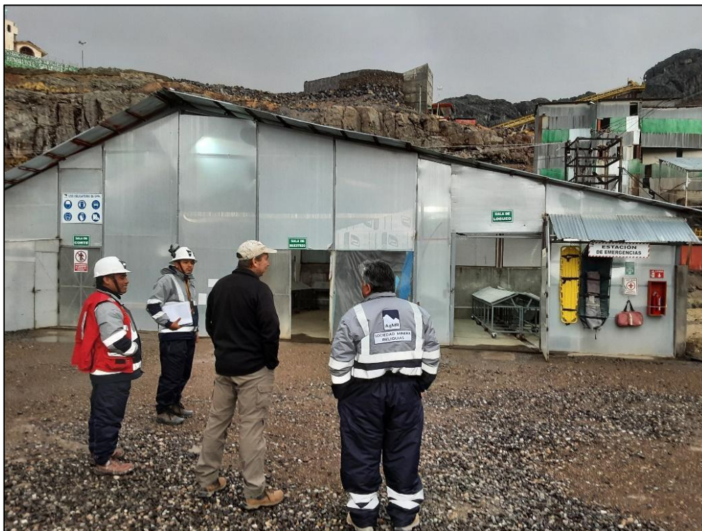
Figure 12.1 Qualified Persons from RREMIN carried out an inspection of the Reliquias Mine facilities in coordination with the SMR staff, here pictured in the drill core storage and logging areas.
