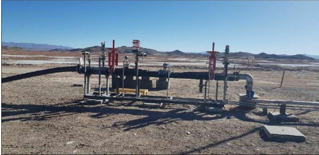
Figure 13-2 - Production Well SVWP21-02.
