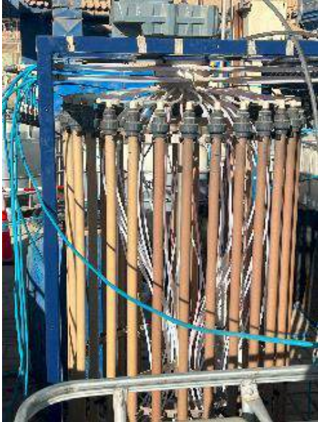
Figure 13-10: Cobalt Loading onto BPA resin.
