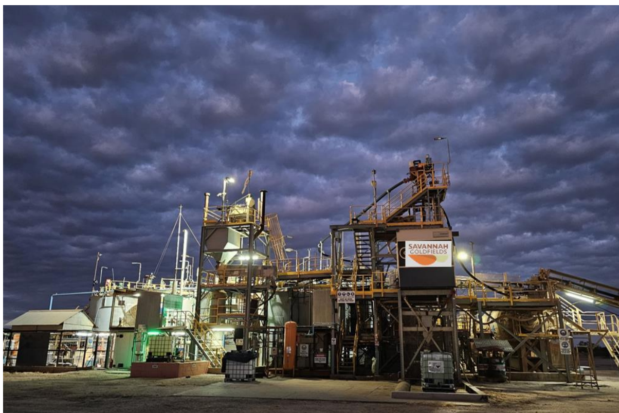
Georgetown Processing Plant
