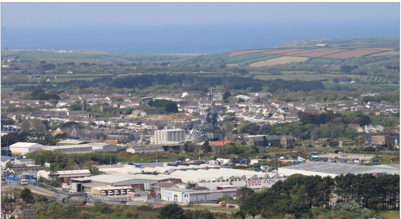
Figure 5.3 Photograph of the NCK headframe
