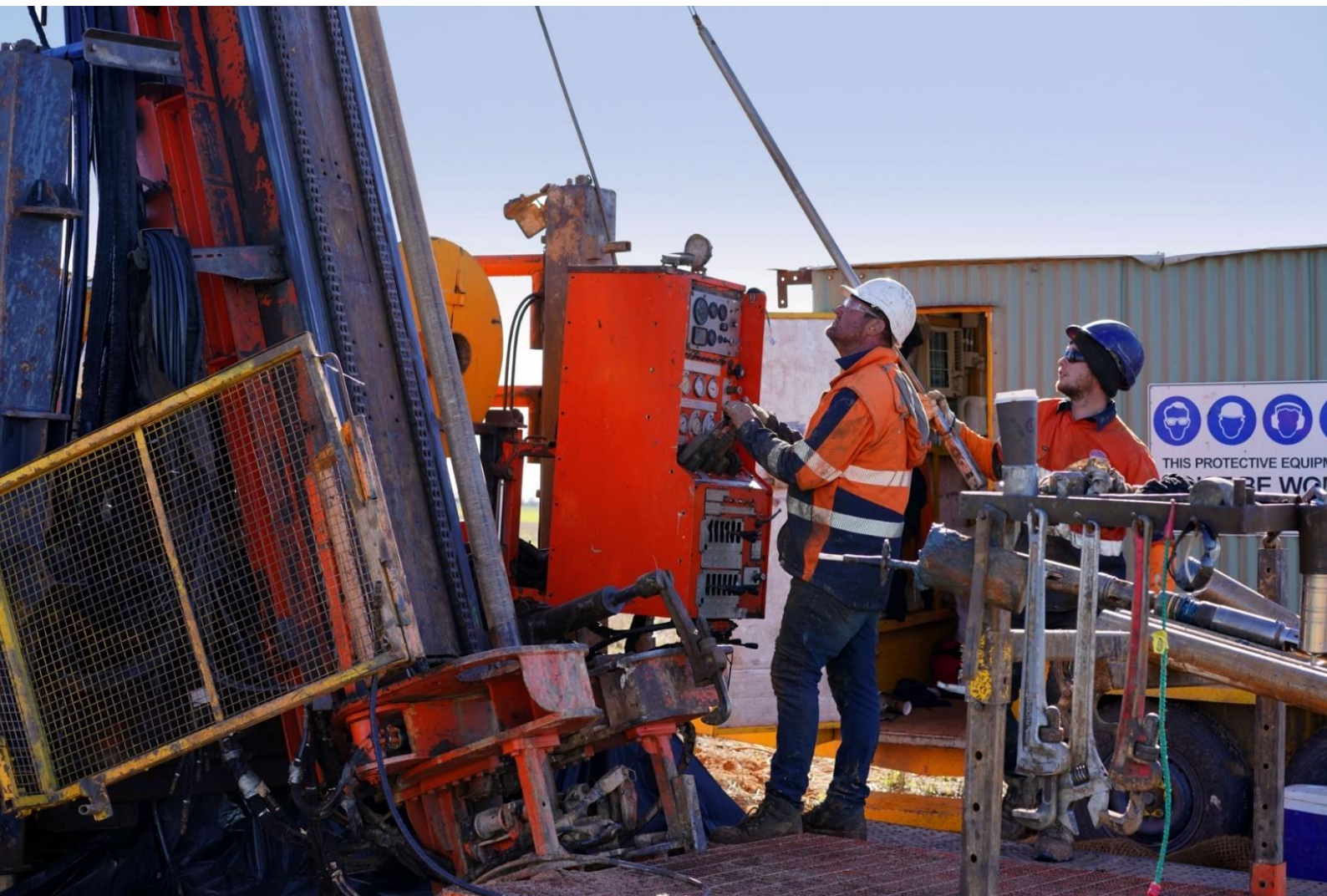
▼ Photo 7: Diamond core drilling at Alford East
