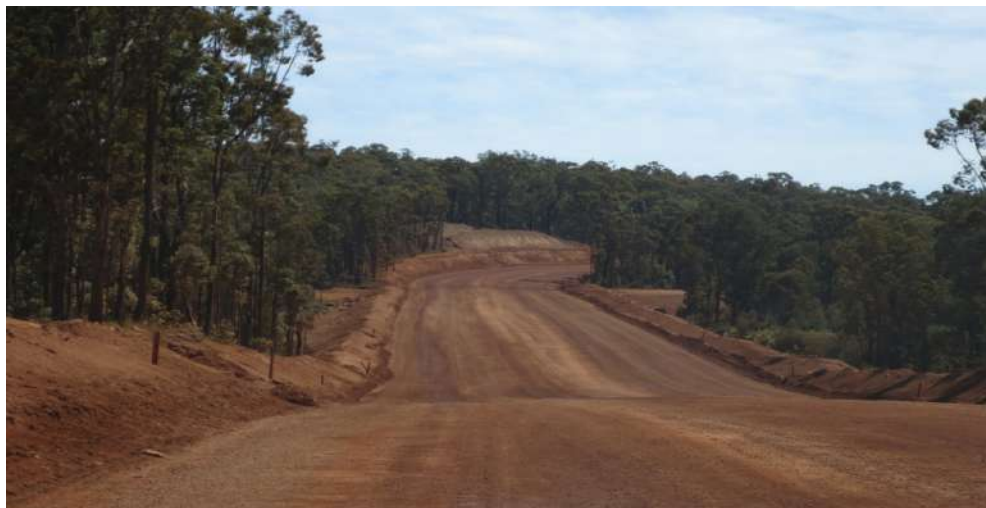
Figure 13-5: Haul Roads with Berms (SLR, 2021)
