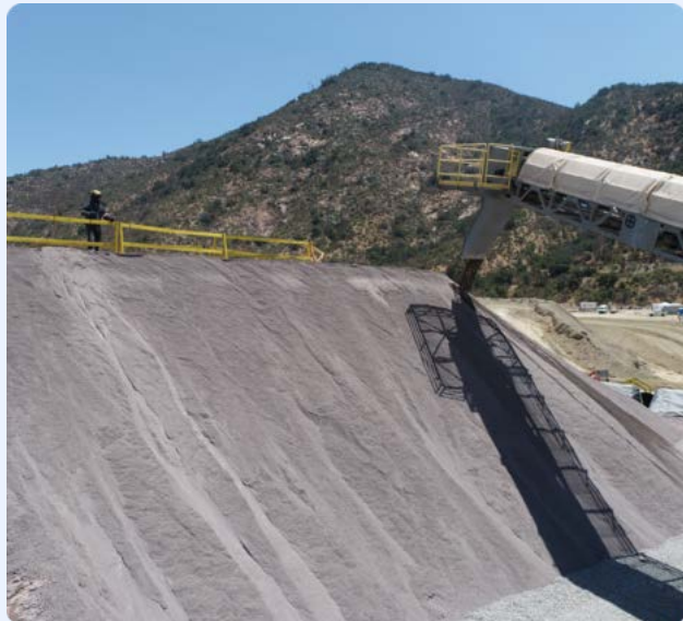
Stacker operator loading sand onto the SandLix™ prototype heap at El Soldado.
