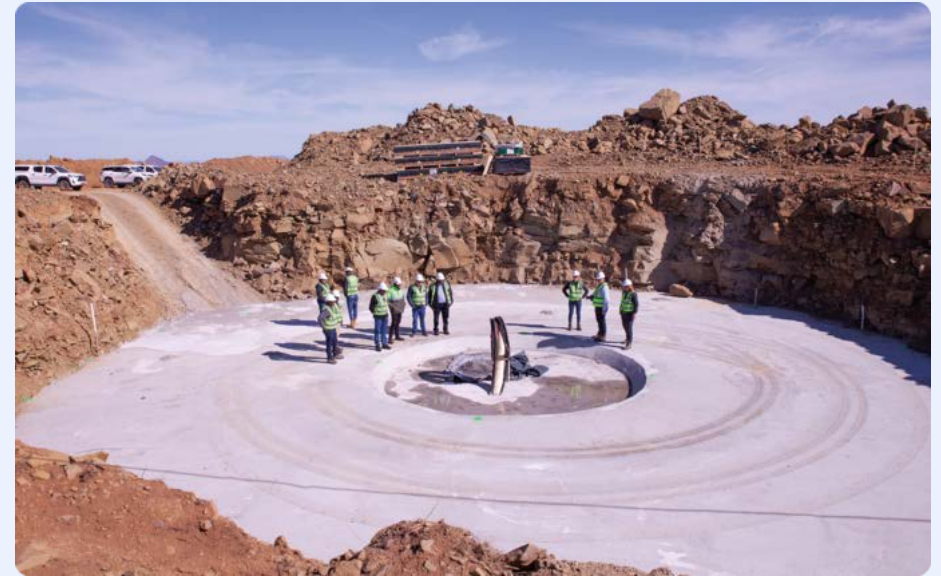
Site visit to the Hartebeesthoek Wind Farm in South Africa that forms part of the Koruson 2 (K2) cluster.
