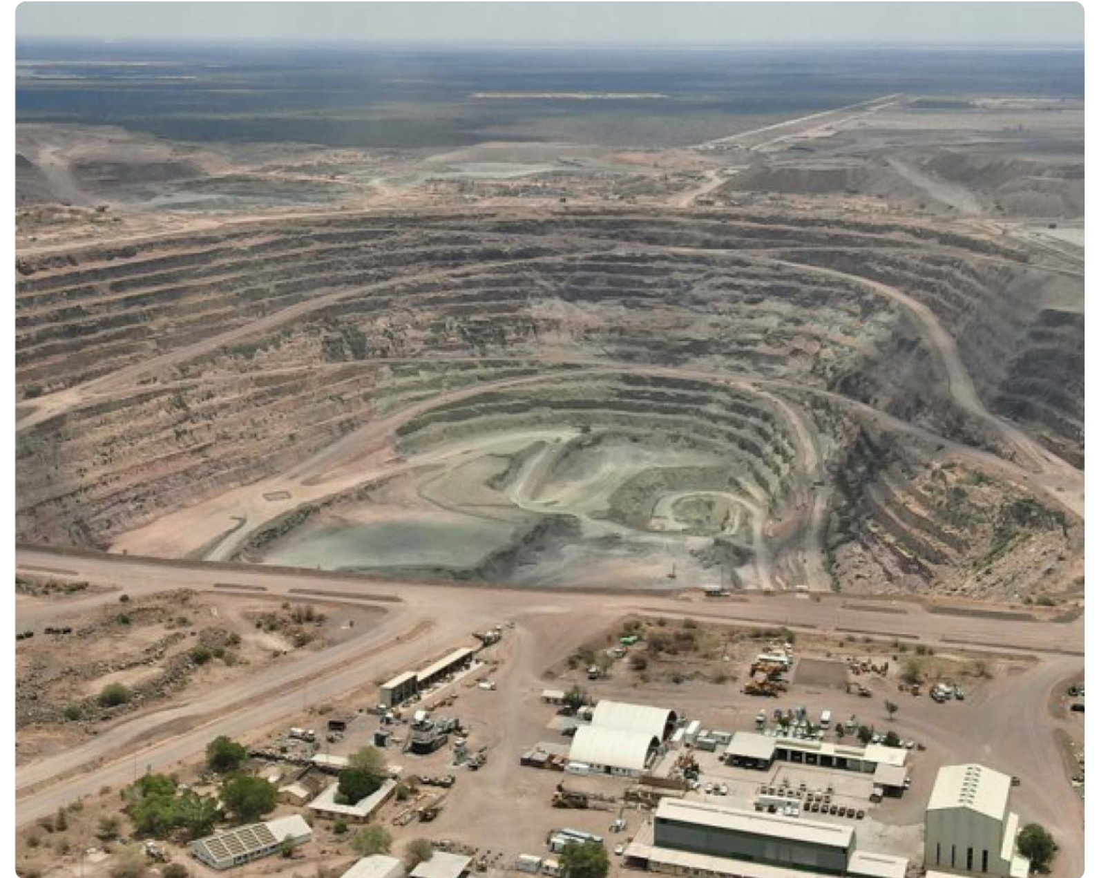
Aerial view of the Orapa diamond mine in Botswana, looking north.
