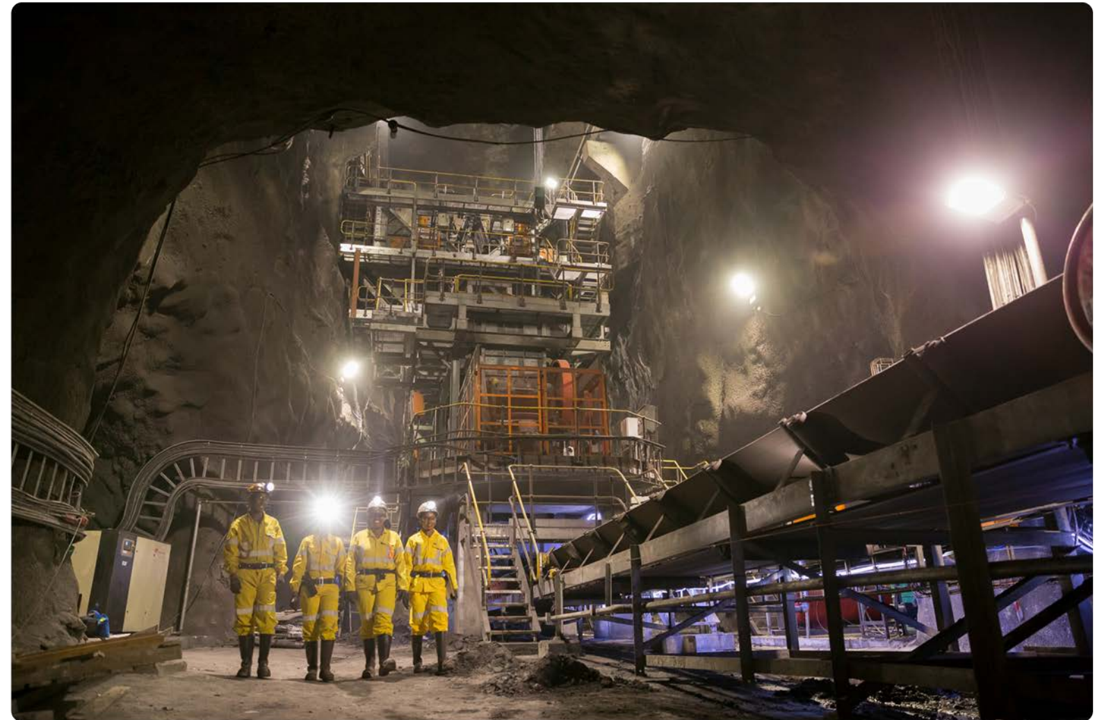
Underground crusher station, Wessels mine, South Africa.
