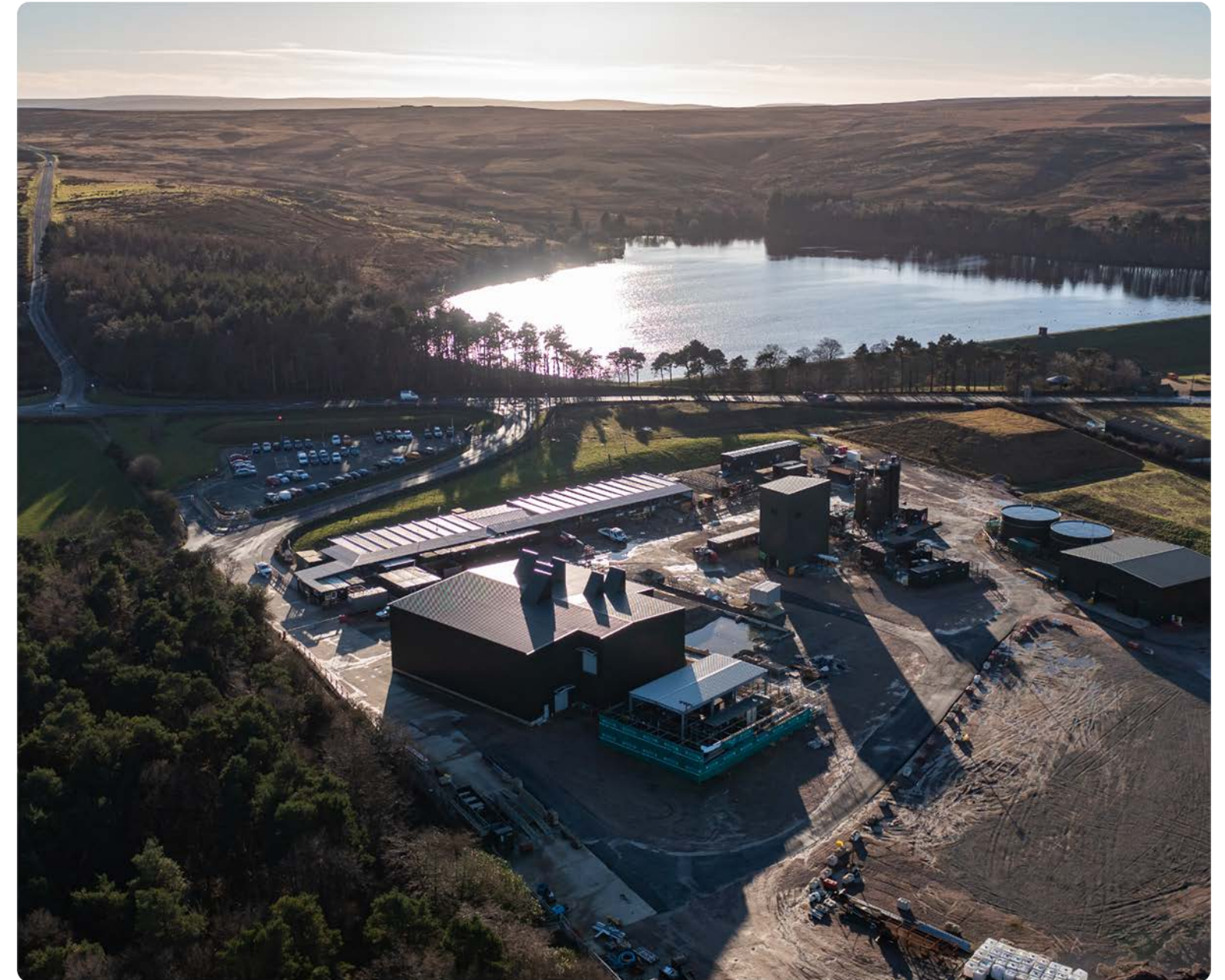
Woodsmith project infrastructure, Lockwood Beck Tunnel access shaft.
