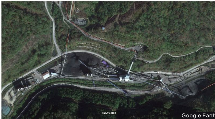
Figure 15-2: Bandmill Preparation Plant
