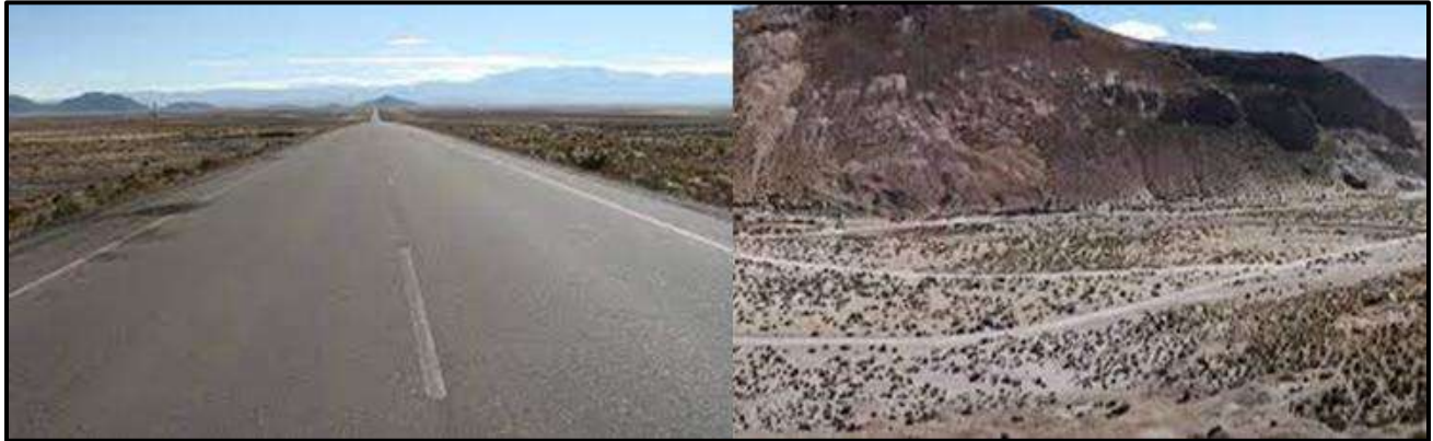
Figure 18-1 Paved Road and Secondary Road to Carangas Project
