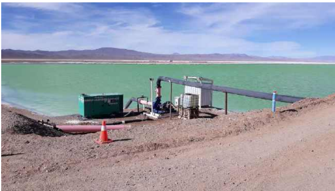
Figure 17.6 Evaporation Ponds – Transfer Pump Station
