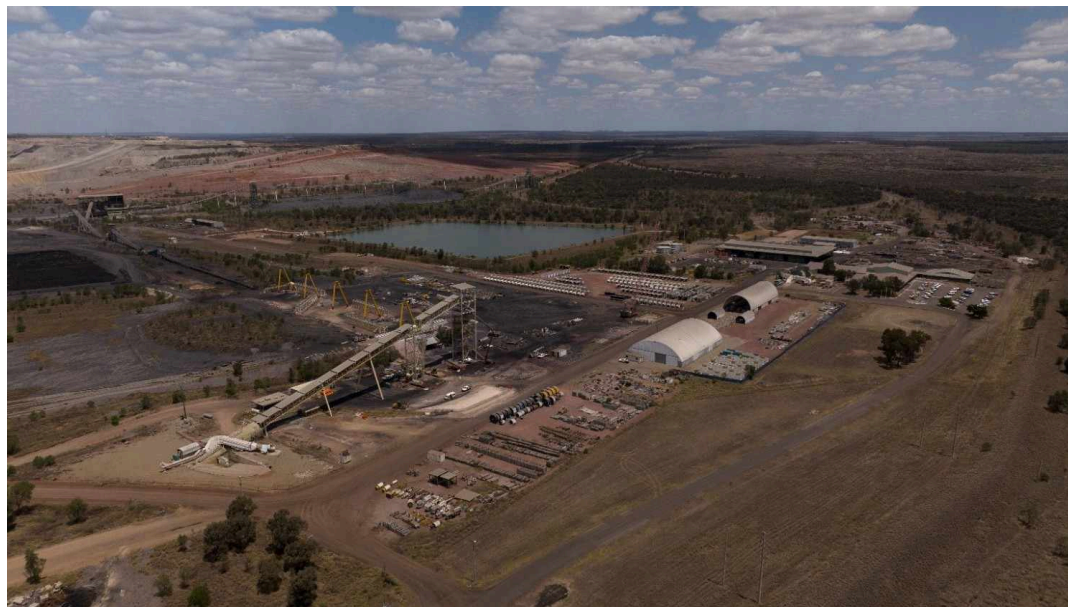
Figure 15-3. Centurion Surface Infrastructure
