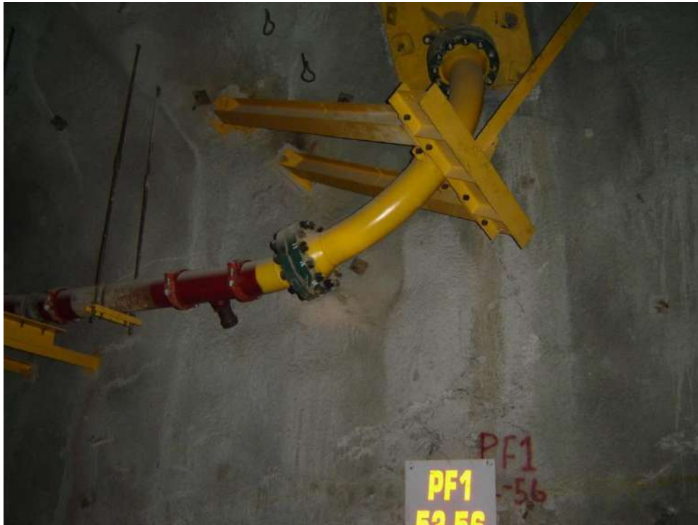
Figure 16.20 – Typical Borehole to Level Piping Connection Configuration
