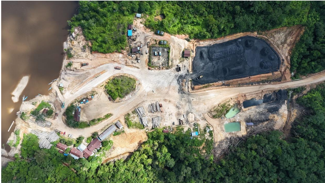
Temporary Krajan Jetty Facilities
