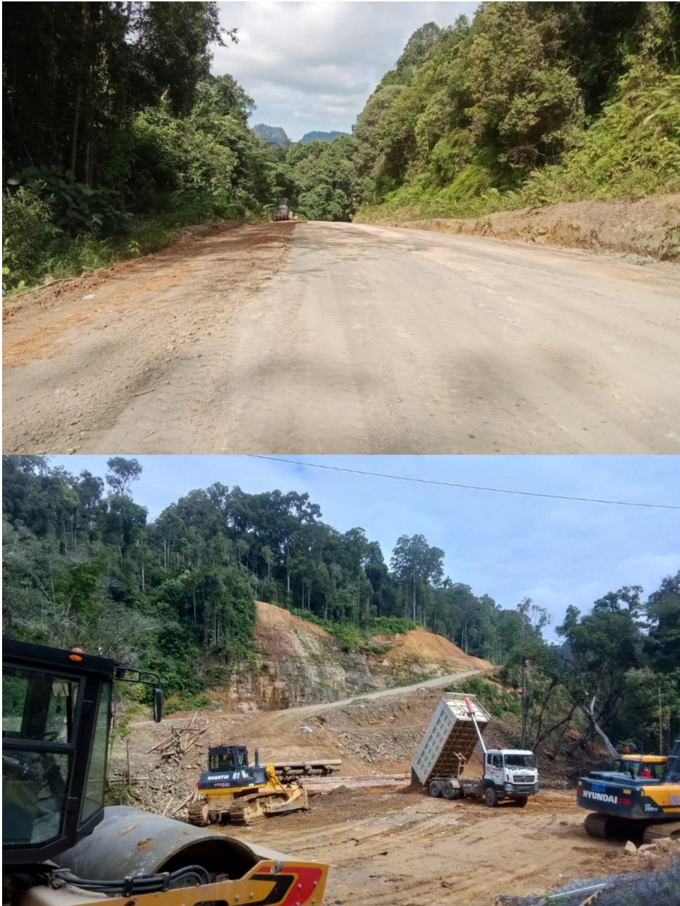
Road & Bridge Construction from Pit 3 to KM52
