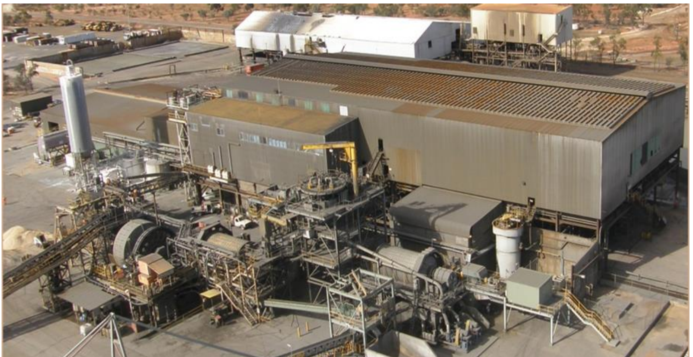
Figure 7: Endeavor Mine Processing Plant
