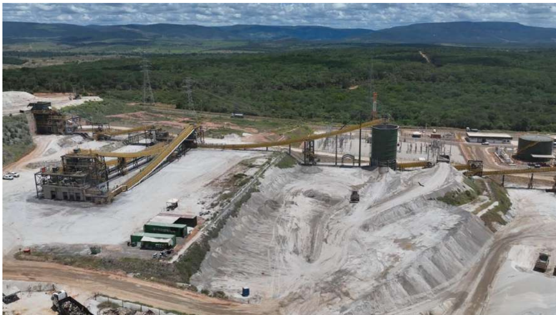
Figure 17-4: Sigma Primary Crushing Facility and Crushed Ore Bin
