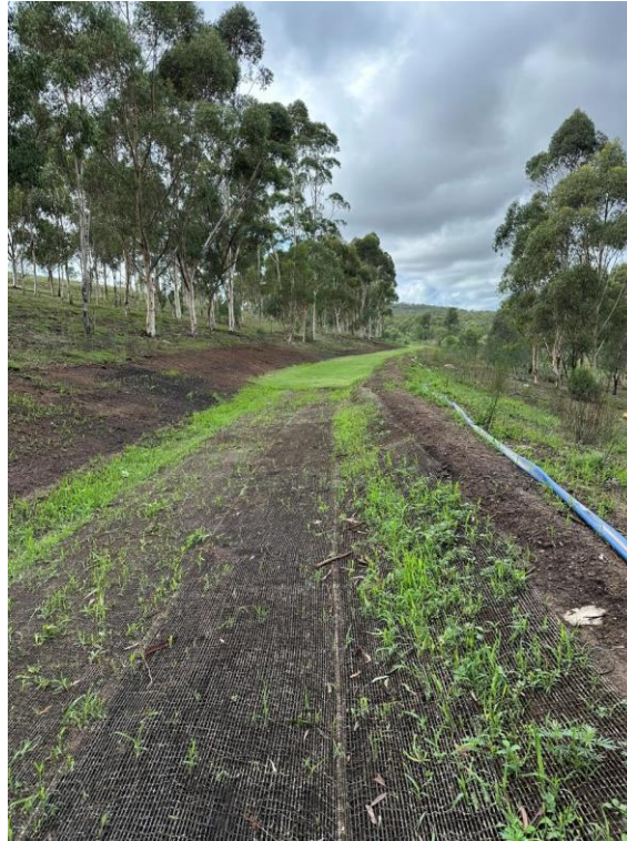
Figure 8-4- Jute mesh and vegetation establishment at WOOP Dump
